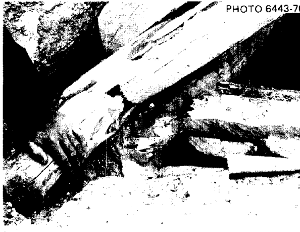
Fig. 6.5. Broken pole of triangular door seat. This pole was broken by differential movements of the earth mounded over the shelter. The man's hand rested on the unbroken hinge pole.
